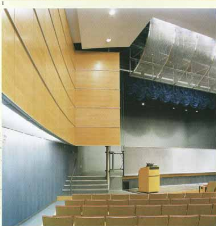
Freeman extended the original stage—only 15 ft deep—with a 6-ft apron on lifts. In the raised position (1), the stage accommodates performances. Lowered, it puts lecturers close to students (3). The
